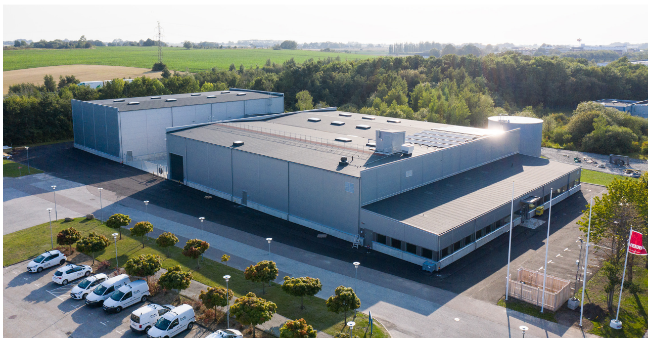
In the fourth quarter of 2020, voestalpine Böhler weldCare AB moved in to an entirely new production facility of 4,300 m 2 at Stenåldern 7 in Fosie, Malmö. Voestalpine is leasing the property on a 15-year lease.
