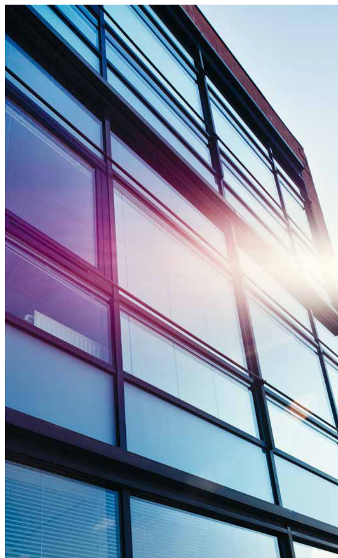
Lautrupvang 1 in Ballerup, Denmark.
